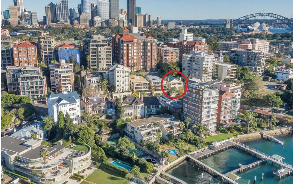
subject site shown in context of Elizabeth Bay
